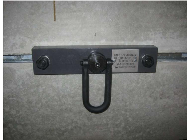
THE STRUT RIGGING PICK POINT HAS A WLL OF 2,000 LBS VERTICAL AND 1,000 LBS IN ANY DIRECTION AND CAN BE INSTALLED ON ANY STRUCTURE THAT HAS PRE-INSTALLED UNISTRUT OR SIMILAR STRUT TRACK. THIS RIGGING PICK POINT ATTACHES DIRECTLY TO THE STRUT TRACK.
